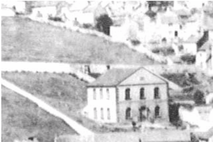
This is how the Chapel looked before the renovation.
